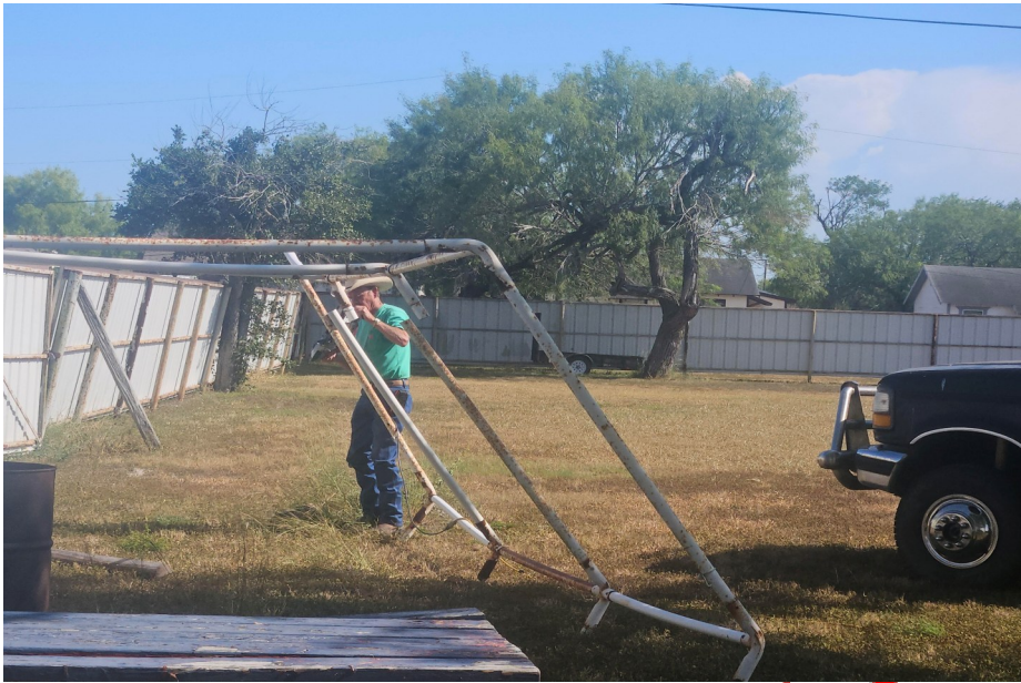
Forrest Lanmon cutting down the old rusty canopies in the backyard.
