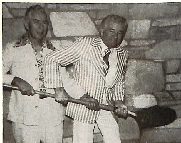
SANTA MARIA, CA. Est. Lead. Kt. Ben Del Mastro (left) and then-ER Bill McDaniel broke ground for a new lodge room at Santa Maria, CA, Lodge. Scheduled for completion in June, the room will have permanent seating for 260 persons.
