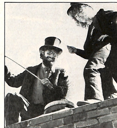
Marty and Kathy Kaylor work to clean out a chimney and make it fire-safe.
