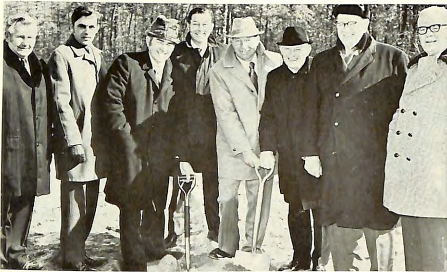
A GROUNDBREAKING ceremony was held recently for Brick, N. J., Lodge's new home. Taking part in the ceremony were (from left) Esq. LeRoy Wutsch, building chairman; John Harvey, Brick Township chairman; ER James Lennon; Est. Lead. Kt. Frank Altomose; Jack Edwards, building contractor; Trustees Chairman Joseph Reilly; DDGER Floyd Gray, and PSP Edward Hanlon.
