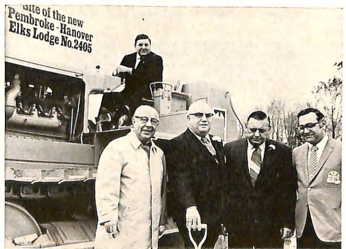
A BULLDOZER was on hand and ready to continue what the groundbreaking ceremony started for the construction of the new Pembroke-Hanover, Mass., Lodge home. Dignitaries taking part in the ceremony included (from left) Grand Trustee W. Edward Wilson; ER Howard F. Levings; Charter ER Theodore S. Kaiser Sr.; DDGER Ambrose C. Rondina, and SP Donald A. Podgurski (seated on bulldozer).
