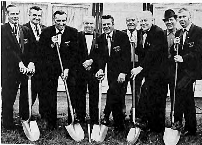
SAUGUS, Massachusetts, Lodge recently broke ground for its new lodge home, a $200,000 structure which will be completed this spring. The ceremony was led by ER Frederick Erickson with DDGER Alfred Fisher of Lynn Lodge assisting. Participants were (from left) Tiler Russell Fratus; Trustee Richard MacLean; Est. Loyal Kt. Stanley Belyea; Trustee Michael McCormick; ER Erickson; Charter Member Robert DeLouis; DDGER Fisher; Trustee James Hogan, and Est. Lect. Kt. Richard Stevens.
