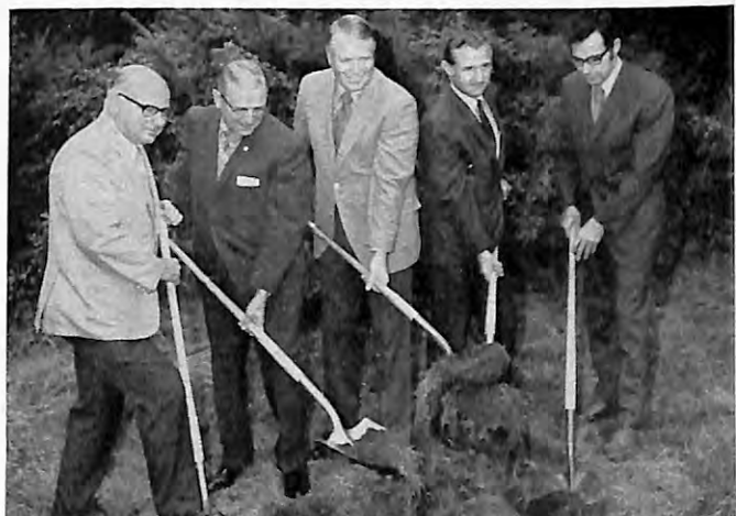
DIGGING IN at the groundbreaking ceremony for the new Kirkland-Bellevue, Wash., Lodge home is this group of distinguished officials. (From left) ER Joe Morell; PGER Frank Hise; Kirkland Mayor Bill Woods; Redmond Mayor S. L. Young and Bellevue City Councilman Dick Foreman joined in officially beginning the construction project that will be completed this spring.
