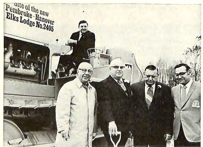
A BULLDOZER was on hand and ready to continue what the groundbreaking ceremony started for the construction of the new Pembroke-Hanover, Mass., Lodge home. Dignitaries taking part in the ceremony included (from left) Grand Trustee W. Edward Wilson; ER Howard F. Levings; Charter ER Theodore S. Kaiser Sr.; DDGER Ambrose C. Rondina, and SP Donald A. Podgurski (seated on bulldozer).
