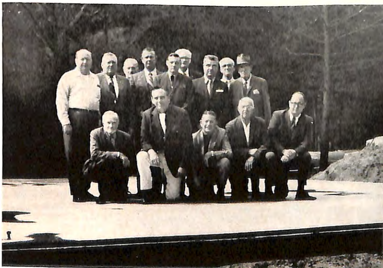
JACKSON, Mississippi , Lodge members gathered to inspect the foundation on which the new lodge home will be built. ER Earl Dimitry Jr. (right) leads the lodge which is growing in members and now in accommodations.
