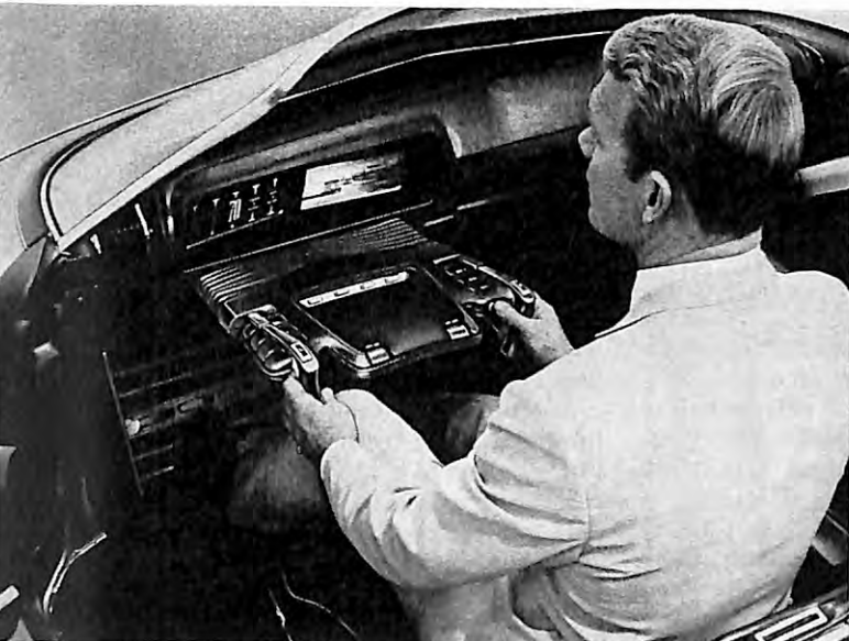
Chrysler's 300X research car (above) replaces conventional steering wheel with light-action hand grips.
