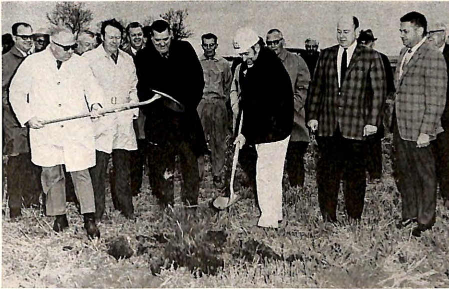
THE FIRST SHOVEL of earth was turned by Michael Kurtz (center) of Michael Kurtz Construction, Inc., at recent groundbreaking ceremonies for the new $430,000 Devils Lake, N.D., Lodge home. Tom Goulding, chairman of the building committee, also participated. ER Kenneth Thompson and Trustees Chairman Les Nyhus were among those present.
