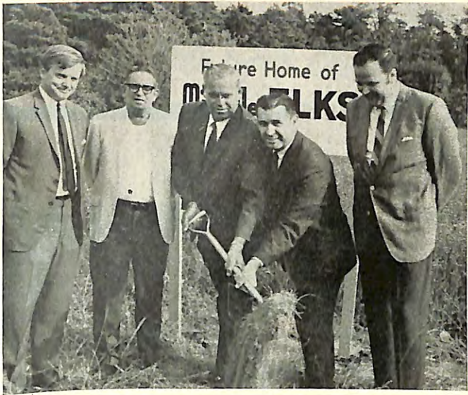
SHOVELING the first spadeful of earth during a recent ground-breaking ceremony for the new Millville, N. J., Lodge quarters are ER John Eller (center) and Millville Mayor Rulon Peek (second from right). The new home, 68 by 110 feet, will be built on seven acres of high-density woodland. Watching the proceedings are (from left) Charles Kulp, builder; PER Jesse H. Smith Sr., building committee chairman, and Est. Lead. Kt. Robert L. Keen.
