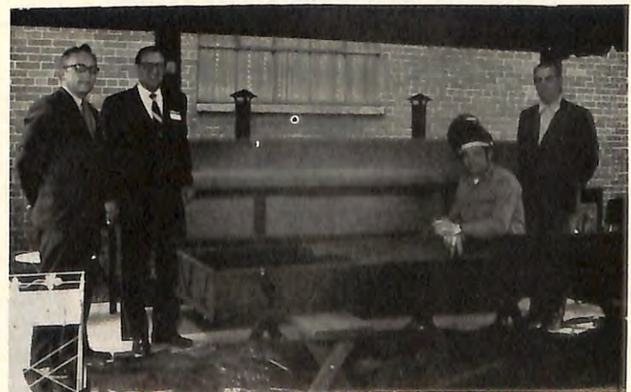
BARBECUED DINNERS will be a specialty at Lancaster, Ohio, Lodge, thanks to three of its members. The plans and construction of the patio and 10-foot grill were completed recently by ER Harry Z. Cook (left), and Brothers Elza Wears (seated) and Harold Feeney (right). Grand Trustee E. Gene Fournace (second from left), of Newark Lodge, was given a special tour while attending the South Central District conference in Lancaster.
