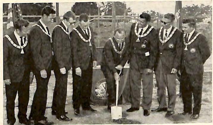
GROUND BREAKING ceremonies for the new $423,000 Valdosta, Ga., Lodge quarters took place recently after five years of planning. The building was designed and will be constructed under the supervision of two Valdosta members. ER Andrew F. Kinard turns the first shovelful of earth, watched by (from left) Est. Lect. Kt. Homer Cody, Esq. Ben Wood, Est. Lead. Kt. Tom Young, Est. Loyal Kt. Harvey Shipman, Secy. Curtis P. Melton, In. Gd. Robert Pinkston, and Chap. Durwood Lewis.
