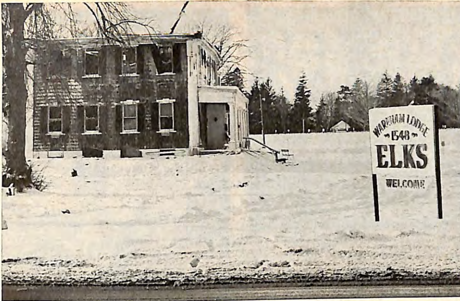
Ice-encrusted, Wareham, Mass., Elks' fire-blackened lodge building bears mute witness to the blaze which ended its many years of activities.
