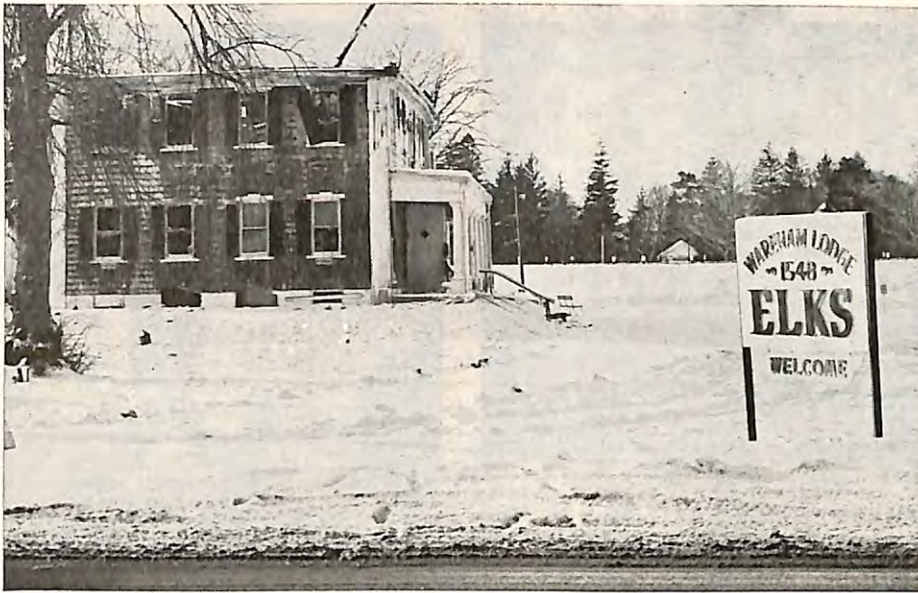
Ice-encrusted, Wareham, Mass., Elks' fire-blackened lodge building bears mute witness to the blaze which ended its many years of activities.
