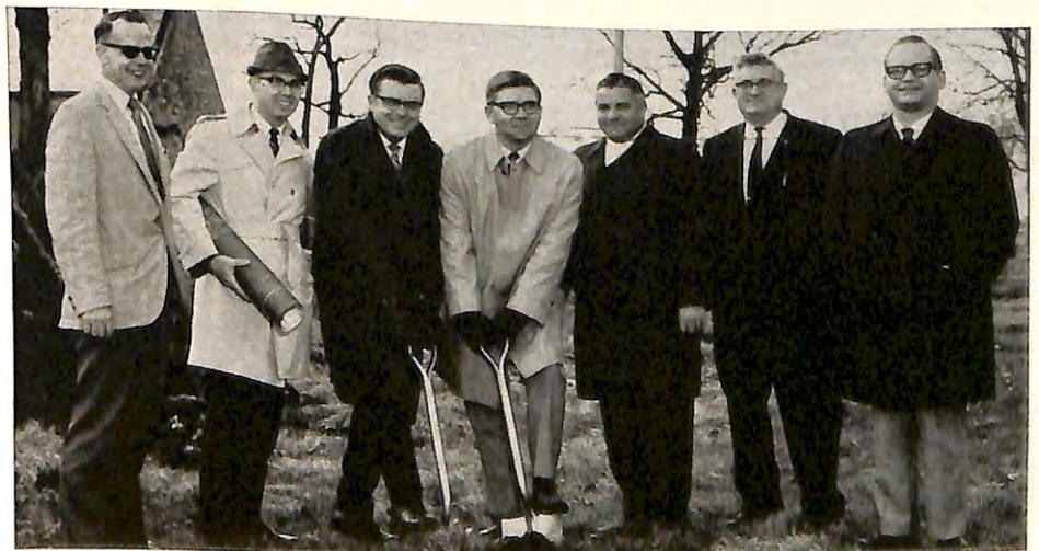
TURNING the first spadeful of earth during groundbreaking ceremonies for their new quarters in Kankakee, Ill., are Kankakee ER Wayne L. Jefferson (third from left) and Est. Lead. Kt. Gene Phillips. Witnessing the event are (from left) Est. Loyal Kt. Tommy Brown; Roline Moline, architect; Norm Felesena, contractor; lodge Trustee Winston Quick, and In. Cd. Roger Benson. The new building boasts an 18-hole golf course.
