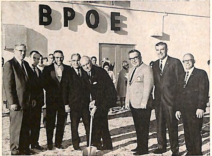
TURNING the first spadeful of earth during groundbreaking ceremonies at North Palm Beach, Fla., Lodge is Florida SP and Dr. R. Lamar Johnston, Vero Beach, as a group of dignitaries present for the occasion bear approving witness. Admiring Brother Johnston's technique are (from left) DDGER George McConnell, Lake Worth; North Palm Beach PER Carl Vaughn, building committee chairman; Brother Leonard L. Miller, in charge of construction arrangements; PGER William A. Wall; North Palm Beach ER Richard Gamache; PDD Robert Grafton, Riviera Beach, and VP Carl J. Hartman, a member of North Palm Beach Lodge.
