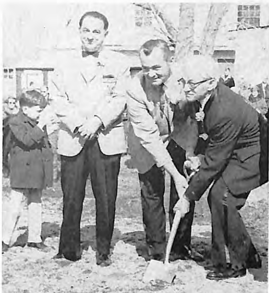
GROUNDBREAKING CEREMONIES for Westbrook, Conn., Lodge's new home commence as one of the 20-year-old lodge's original founders and its first Exalted Ruler, Brother Anthony Gasparini (right), and his son, immediate PER Clifford R. Gasparini, wield the shovel. Trustees Chairman Sylvester Dente looks on. Among the Elks dignitaries attending the ceremonies was Grand Treas. Edwin J. Maley, of New Haven Lodge, who addressed the gathering.
