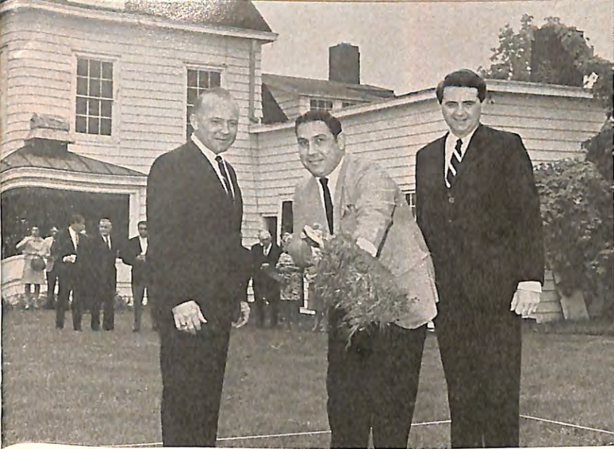
A BIT OF OLD SOD is shoveled by Mount Kisco, N.Y., ER Salvatore A. Adorno at groundbreaking ceremonies for the lodge's new $500,000 building. Flanking him are DDGER Edward F. Ahneman Jr. (left), a member of Mount Kisco Lodge, and Mayor Henry V. Kensing.
