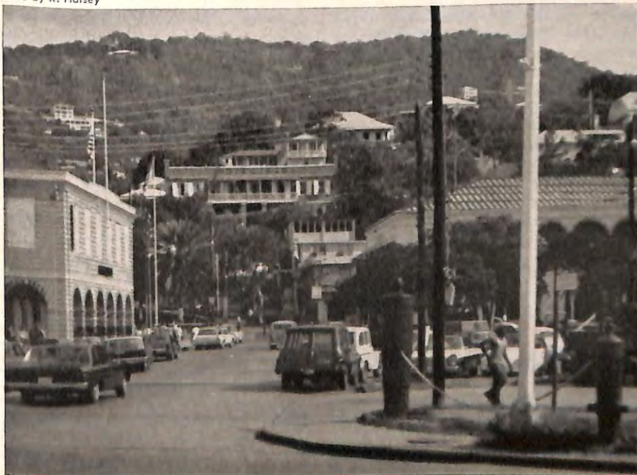
The Hotel 1829 stands on a hill (background) overlooking the town of Charlotte Amalie on the island of St. Thomas. This street is characteristic of those on the islands.
