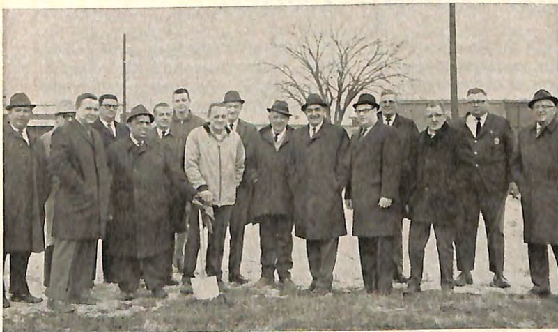
ROCHESTER, New Hampshire, Elks break ground for a new $162,000 building. Lodge members and building committeemen and guests attending the ceremony are: (from left) Richard Rouleau, contractor; Henry Euler, architect; PER Frank D. Callaghan Jr., trustees chairman; Brother Robert Carignan; Trustee George Nadeau, building chairman; Brother Ronald Tebbetts; Brother Carl Stevens; ER Leon Lachapelle; PER Dennis E. Brennan; PDD Lucien Langelier; Treas. Joseph Zuromskis; PER Joseph D. Rigazio; Brother Winston Nichols; PER George A. Lachapelle; Trustee Leland Waterhouse, and Secy. Berton D. Bryant.
