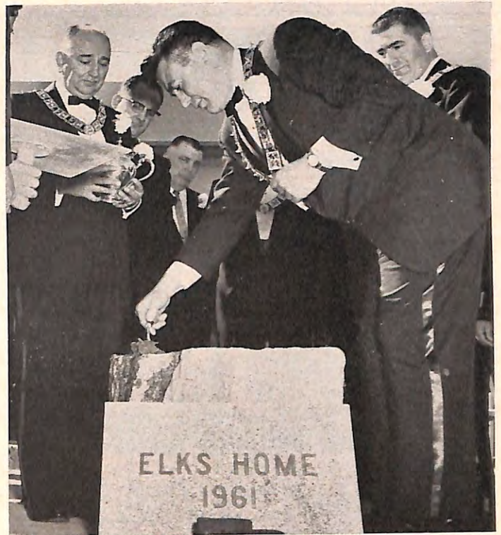
RENO, Nevada, Lodge's E.R. Albert Solari applies mortar in the cornerstone laying for the lodge's new home. Others include Est. Loyal Knight Don Rose, Past Grand Exalted Ruler H. R. Wisely, background, and Chaplain Louis Capurro, far right.
