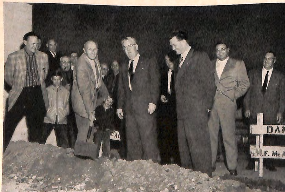
VICTORVILLE, California, Lodge's groundbreaking for the addition to its home was handled by guest of honor State Pres. Guy A. Daniels, second from left. Others pictured in the foreground include, left to right, R. John Blesch, Jr., architect for the 2,300 sq. foot addition, E.R. Edw. A. Rodeman and D.D. Robert A. Kennepohl. The new building, the third expansion for this lodge in the eight years of its existence, will provide modern kitchen facilities and added recreation areas for its members.
