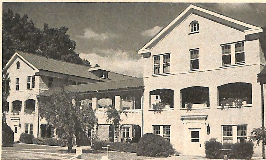
Residence cottages, surrounded by trees, shrubbery and well-kept lawns, give the National Home an atmosphere of comfort, privacy and serenity.
