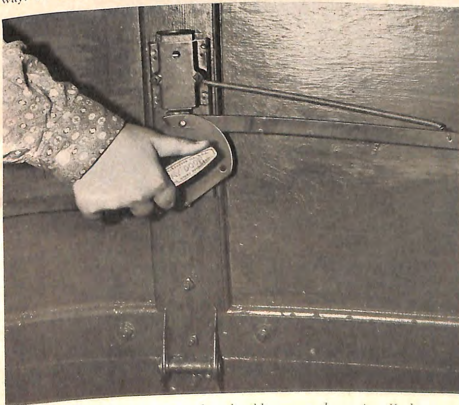
A broken latch spring is easily replaced by a screen-door spring. Hook at least two turns of it into a hole in a latch bar and the same over a bolt in the housing. Make sure both ends are securely engaged.
