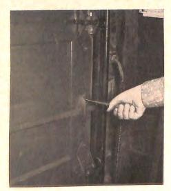
When the latch or bar won't enter its socket, first make sure some obstruction isn't preventing the door from going down all the way. Then adjust guide by loosening screws as shown and tapping it into alignment.
