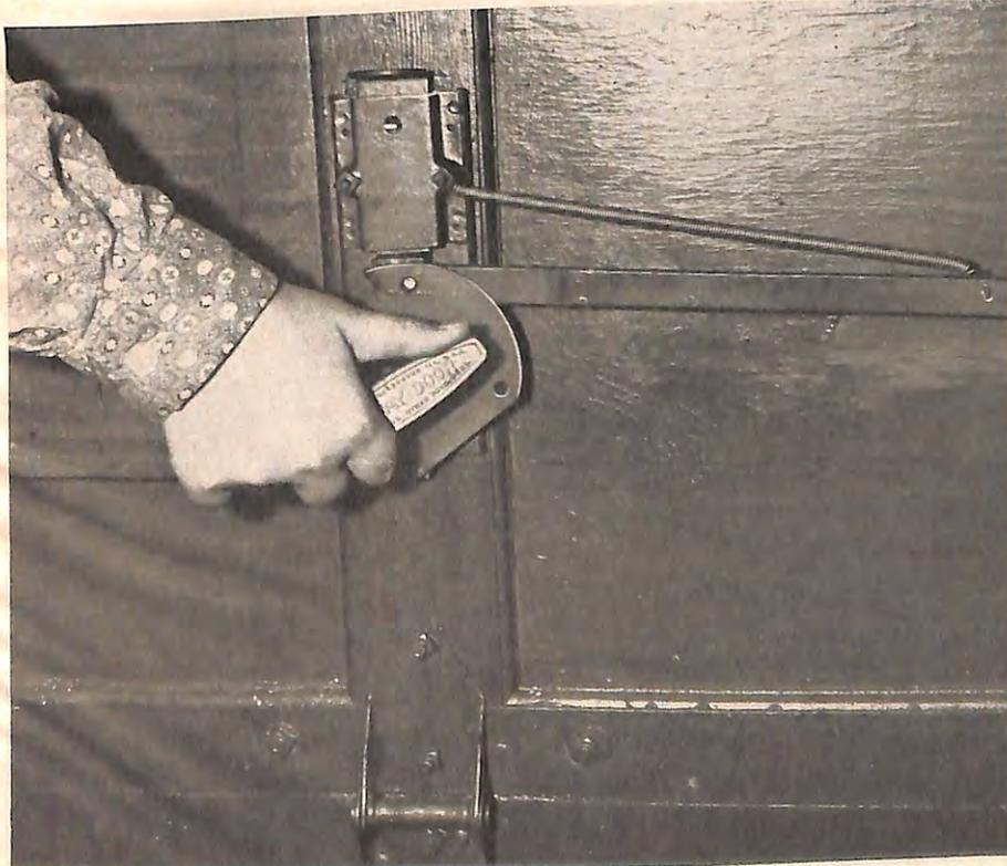
A broken latch spring is easily replaced by a screen-door spring. Hook at least two turns of it into a hole in a latch bar and the same over a bolt in the housing. Make sure both ends are securely engaged.
