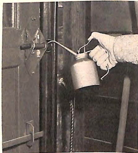
Sectional doors have ten rollers like this one. Oil them and the hinge pins (which extend to carry rollers) to reduce lifting effort.
