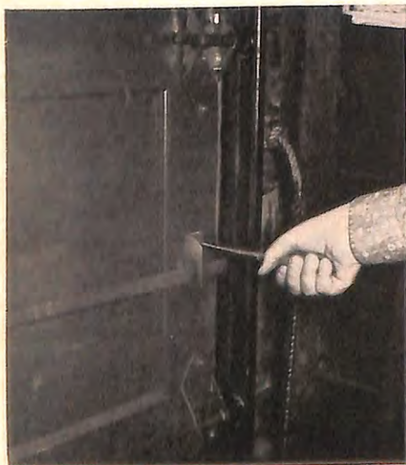
When the latch or bar won't enter its socket, first make sure some obstruction isn't preventing the door from going down all the way. Then adjust guide by loosening screws as shown and tapping it into alignment.
