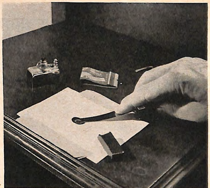
USE A CLEAN FLAME to heat the spatula or knife when applying stick shellac to a gouge or hole. Mask the unmarred surface with paper, and press shellac into the cavity (above, left); holding spatula horizontally (right), build up layers slightly higher than surface.
