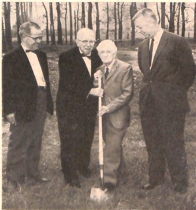
ELWOOD, Indiana, Lodge's new home is now under construction, following the special ground-breaking ceremony in which the lodge's only living Charter Member, P.E.R. Joseph DeHority, an Elk for 65 years and the lodge's first Secy., third from left, was assisted by Past Grand Exalted Ruler Joseph B. Kyle, second from left. Looking on are Special Deputy Robert L. DeHority, left, and E.R. Weldon Shickley.
