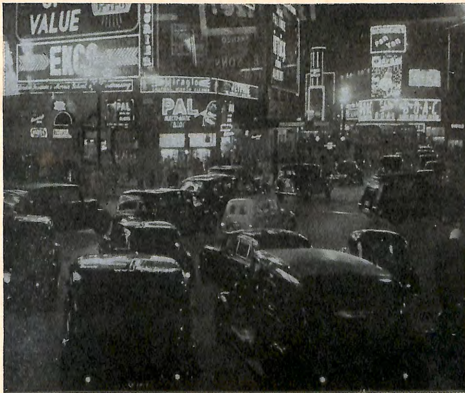
Piccadilly Circus is one of the world's most gaily lit traffic centers—and one of the busiest. Five main streets converge here in the center of West End.
