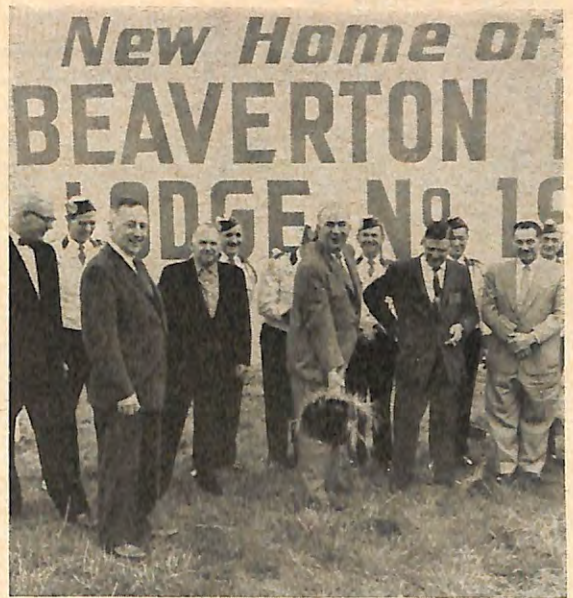
Breaking ground for the construction of Beaverton, Ore., Lodge's new $85,000 home, Mr. Hawkins turns the first spade of soil on April 3, while Exalted Ruler J. D. Stevenson (foreground) and lodge members watch. Target date for completion is August 1.
