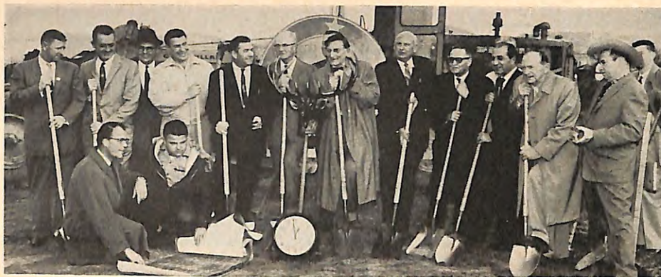
RENO, Nevada, Elks broke ground for their proposed $645,000 home three years to the minute, as indicated by the clock in the foreground, after the lodge lost its home in the tragic explosion and fire of Feb. 7, 1957. Left to right, standing, are Mayor Bud Baker, P.E.R. A. J. Caton, Jr., Est. Loyal Knight F. L. Hill, Inner Guard L. J. Capurro, P.E.R. H. J. Gazin, Treas. P.E.R. A. L. Crocker, E.R. Jack Peters, P.E.R.'s E. P. Caffrey and Vern Hursh, Esq. Tom Johnson, P.E.R. Lino Del Grande, Secy. J. C. Kumle, Toor Root and D. C. Kitselman. Foreground, Elks E. S. Parsons, architect, and J. C. Dillard, contractor. Plans for the home include a swimming pool.
