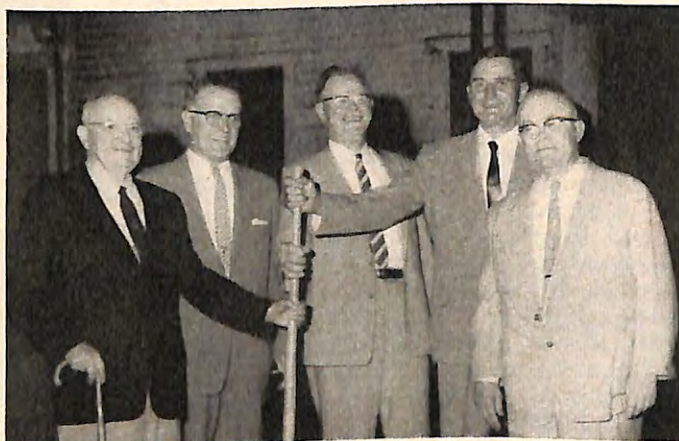
DECATUR, Indiana, Lodge had these officials break ground for its new $65,000 home. Left to right: Charter Member I. A. Kalver, Grand Lodge Committeeman Robert L. DeHority, E.R. George Bair, contractor Cal Yost and State Pres. Leonard Imel.
