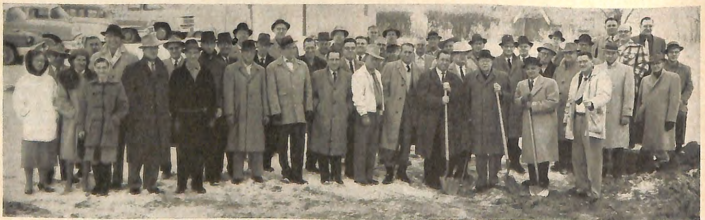
IDAHO FALLS, Idaho , Lodge breaks ground for its $500,000 home. Participating dignitaries included Mayor John B. Rogers, Contractor Golden Wadsworth, Architect C. A. Sundberg, Trustees Chairman P.E.R. B. J. Bybee, the lodge's sole surviving Charter Member Frank Bowman, E.R. Dr. Peter G. Schroeck, P.E.R.'s C. S. Lowrie and John Westergard, Secy. E. C. Moore, Trustee and P.E.R. Robert Jahn and Est. Lead. Knight N. D. Andersen.
