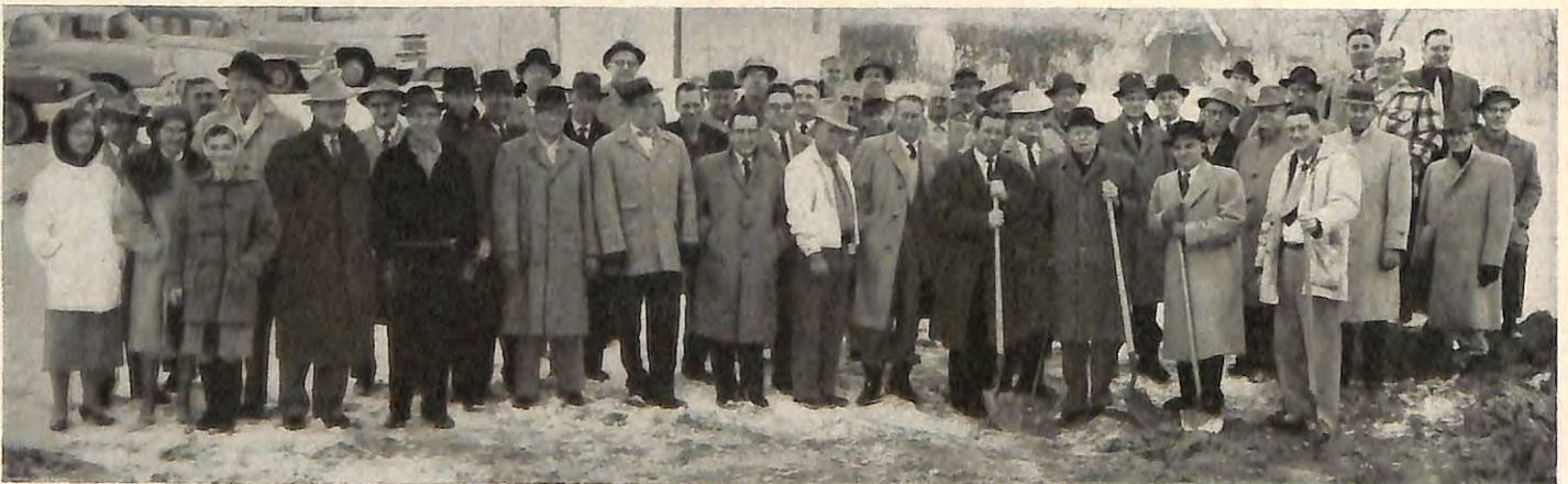
IDAHO FALLS, Idaho , Lodge breaks ground for its $500,000 home. Participating dignitaries included Mayor John B. Rogers, Contractor Golden Wadsworth, Architect C. A. Sundberg, Trustees Chairman P.E.R. B. J. Bybee, the lodge's sole surviving Charter Member Frank Bowman, E.R. Dr. Peter G. Schroeck, P.E.R.'s C. S. Lowrie and John Westergard, Secy. E. G. Moore, Trustee and P.E.R. Robert Jahn and Est. Lead. Knight N. D. Andersen.
