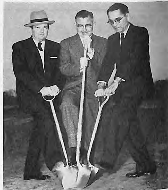
Breaking ground for the Tulsa, Okla., Lodge's $250,000 home and swimming pool are, left to right, D.D. L. A. Wood, retiring E.R. L. R. Hedrick and retiring State Pres. Bert Wysor.
