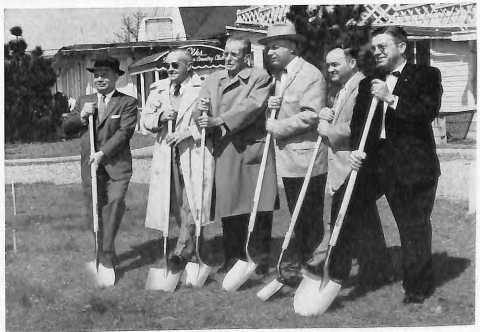
Breaking ground for the $120,000 swimming pool which is being constructed at the Terre Haute, Ind., Elks' Fort Harrison Country Club were, left to right, P.E.R. James J. Jenkins, P.E.R.'s and Trustees Karl Werneke and H. E. Hickman, Trustee and House Committee Chairman John G. Schmidt, Pool Committee Chairman Dr. Byron E. Price and Exalted Ruler Raymond F. Fischer.
