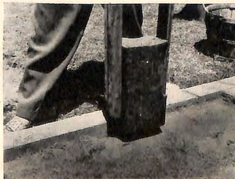
Tamping the sand base insures a firm bed and reduces shifting of paving units.
