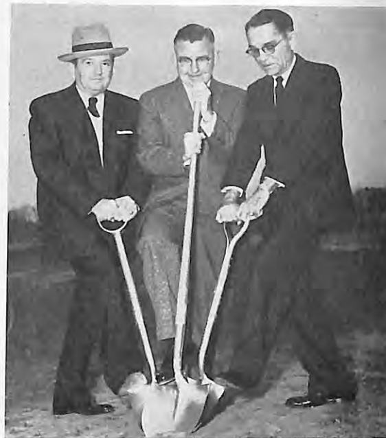
Breaking ground for the Tulsa, Okla., Lodge's $250,000 home and swimming pool are, left to right, D.D. L. A. Wood, retiring E.R. L. R. Hedrick and retiring State Pres. Bert Wysor.
