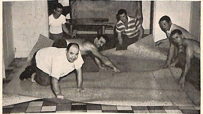
Orlando, Florida, Elks wouldn't "let George do it" when it came to installing the Sandran Floor Covering they had purchased for the Primrose School for Retarded Children. Capably handling the job in true do-it-yourself fashion are A. R. Siler, Leonard Boehm, H. D. Dubler, Adron D. Ratliff, August Engelhardt and Kenneth MacPherson.
