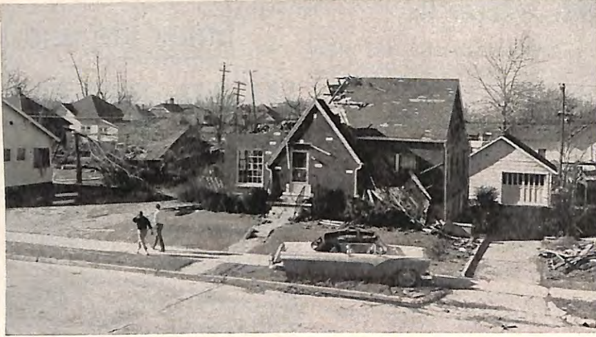
This shattered home shows the tornado damage in Chaffee.
