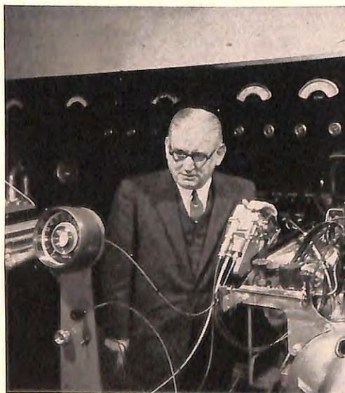
Emlyn Lloyd, Director of Purchasing for Chrysler Corporation, resting his hand on the “Auto-Pilot” speed control device as it undergoes tests in the company’s engineering division laboratories.
