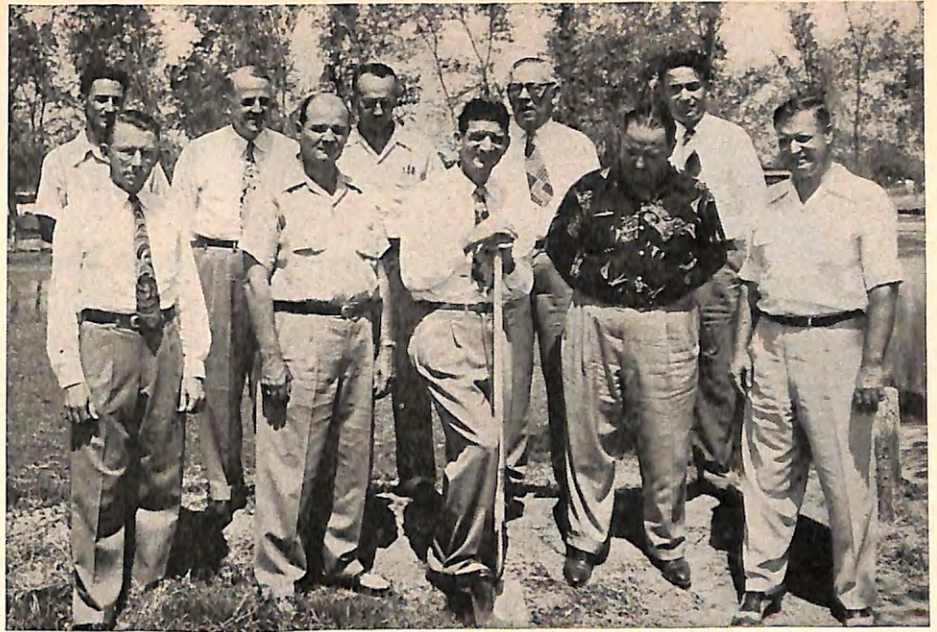
Phoenix, Ariz., Elks break ground for the clubhouse to be erected on a ten-acre plot for the benefit of the Elks and their families, as well as for the Boy Scouts and other local youth groups.
