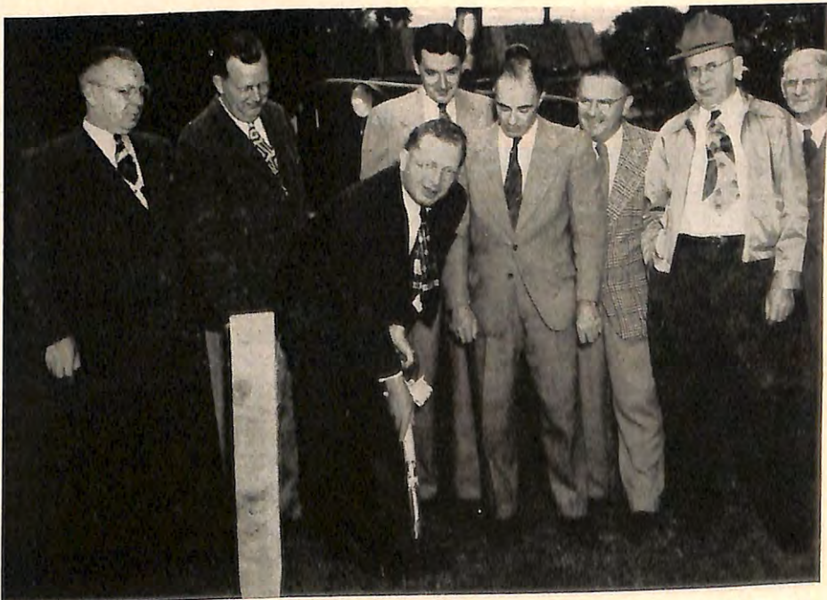
State Supreme Court Justice Robert E. Noonan, P.D.D., turns over the first spade of earth on the site of the $100,000 addition to Batavia, N. Y., Lodge's home. Also pictured are E.R. Vincent R. Callahan and other Elk officials, as well as the building's architect and the contractor.
