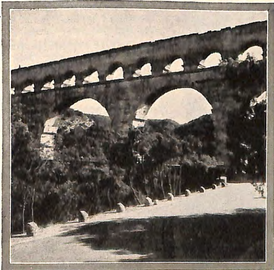
THREE-DECKED AQUEDUCT , built by the Romans about 55 B.C. crosses the river Gard, bringing water 25 miles from the mountains to Nimes. Many interesting excursions radiate from here.
