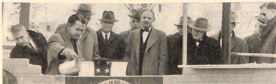
Exalted Ruler Bernard Callahan pours water from a ewer at the cornerstone-laying for the new home of Littleton, Colo., Lodge, as other Elk officials, including D.D. Ralph H. Dial, look on.
