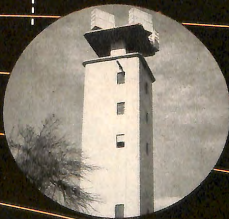
RADIO RELAY TOWER
