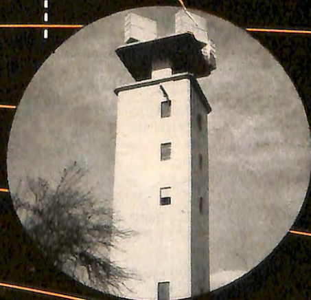
RADIO RELAY TOWER
