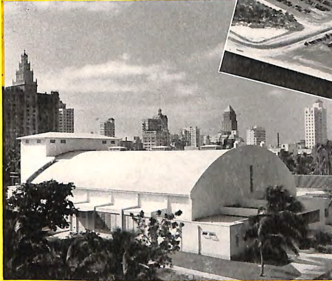
Miami's Municipal Auditorium, where the sessions of the 1950 Grand Lodge Convention will be held, has a capacity of 3,500.
