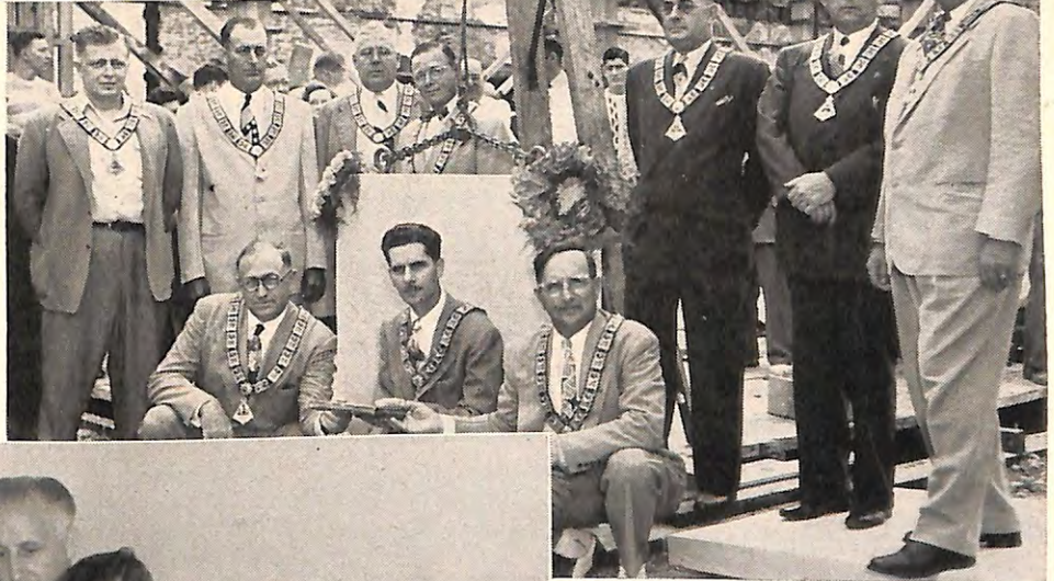
Right: Officers, joined by D.D. Ben L. Rowekamp and P.D.D. Forrest C. Simon, lay the cornerstone for the new home of Piqua, Ohio, Lodge to take the place of the building which was destroyed by fire over a year ago.
