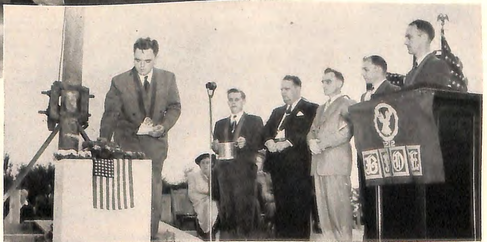
Right: E.R. Robert Ellingen, assisted by his corps of officers of Mendota, Ill., Lodge, conducted the ceremony for the laying of the cornerstone to the city's new hospital.
