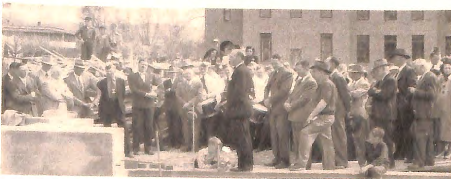
D.D. Oskar O. Lympus stands on the foundation of Hamilton, Mont., Lodge's new home to deliver an address to a large audience as construction was started.
