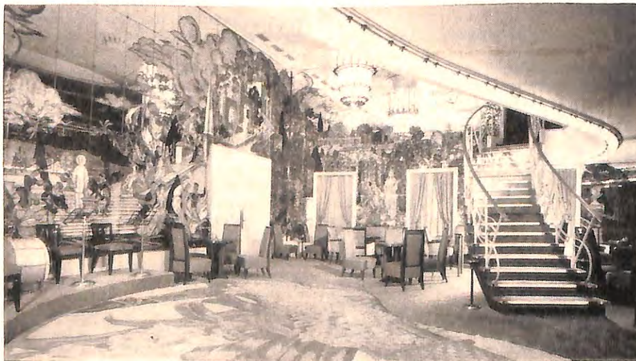
Cabin class salon on the rebuilt Ile de France .
