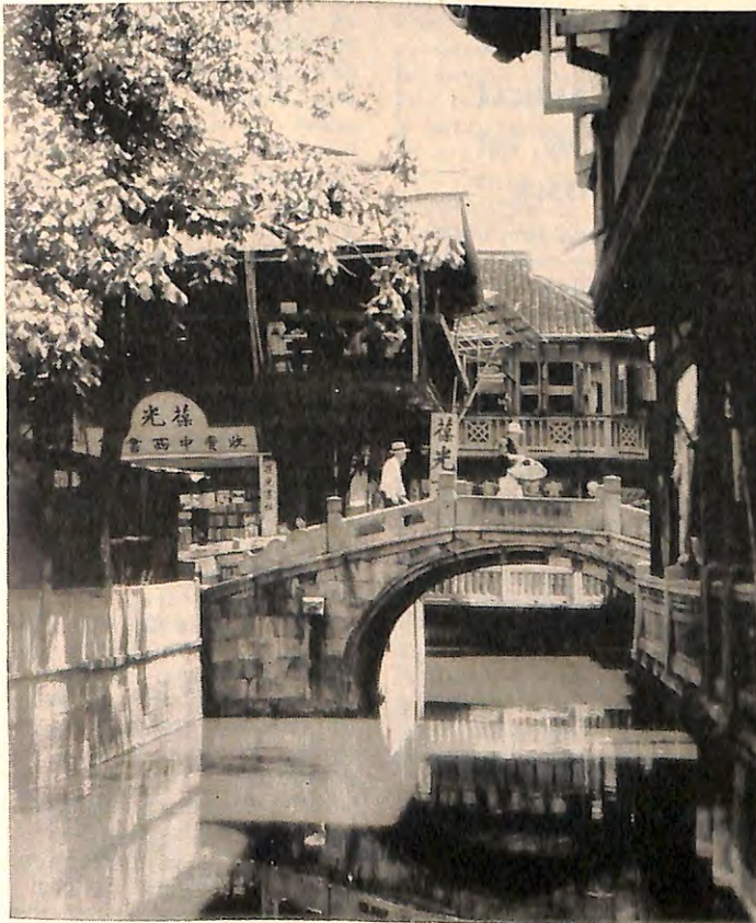
Stone bridge over a canal in the Old City of Shanghai.
