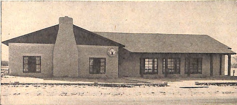
District and national Elk officers, including Past Grand Exalted Rulers Michael F. Shannon and L. A. Lewis, and D.D. R. N. Traver, participated in the dedication of this lovely new home of Hemet, Calif., Lodge. Erected recently at the cost of $50,000, the building already has been the scene of many lodge meetings and social events staged by Hemet Lodge which has been in existence only since April, 1948.
