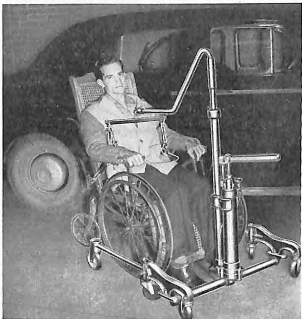
This illustrates the easy method by which Porto-Lift aids the difficult task of transferring a patient from wheel chair to automobile. The use of the single arm, swivel bar, and two wide straps, make for greater comfort to the patient, and eliminates a troublesome job for attendants.
